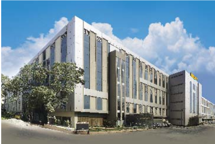
Switchgear Factory, Mumbai
