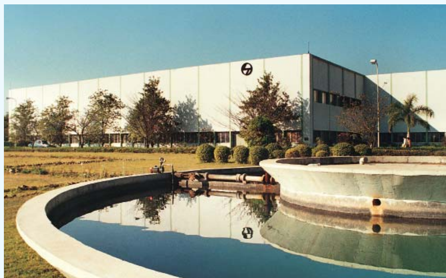
Switchgear Factory, Ahmednagar
