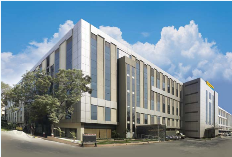
Switchgear Factory, Mumbai
