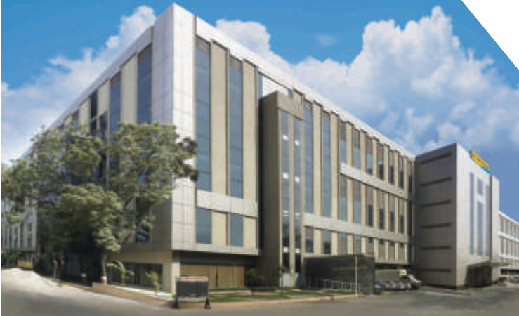
Switchgear Factory, Mumbai
