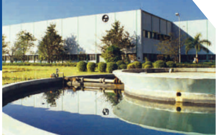
Switchgear Factory, Ahmednagar
